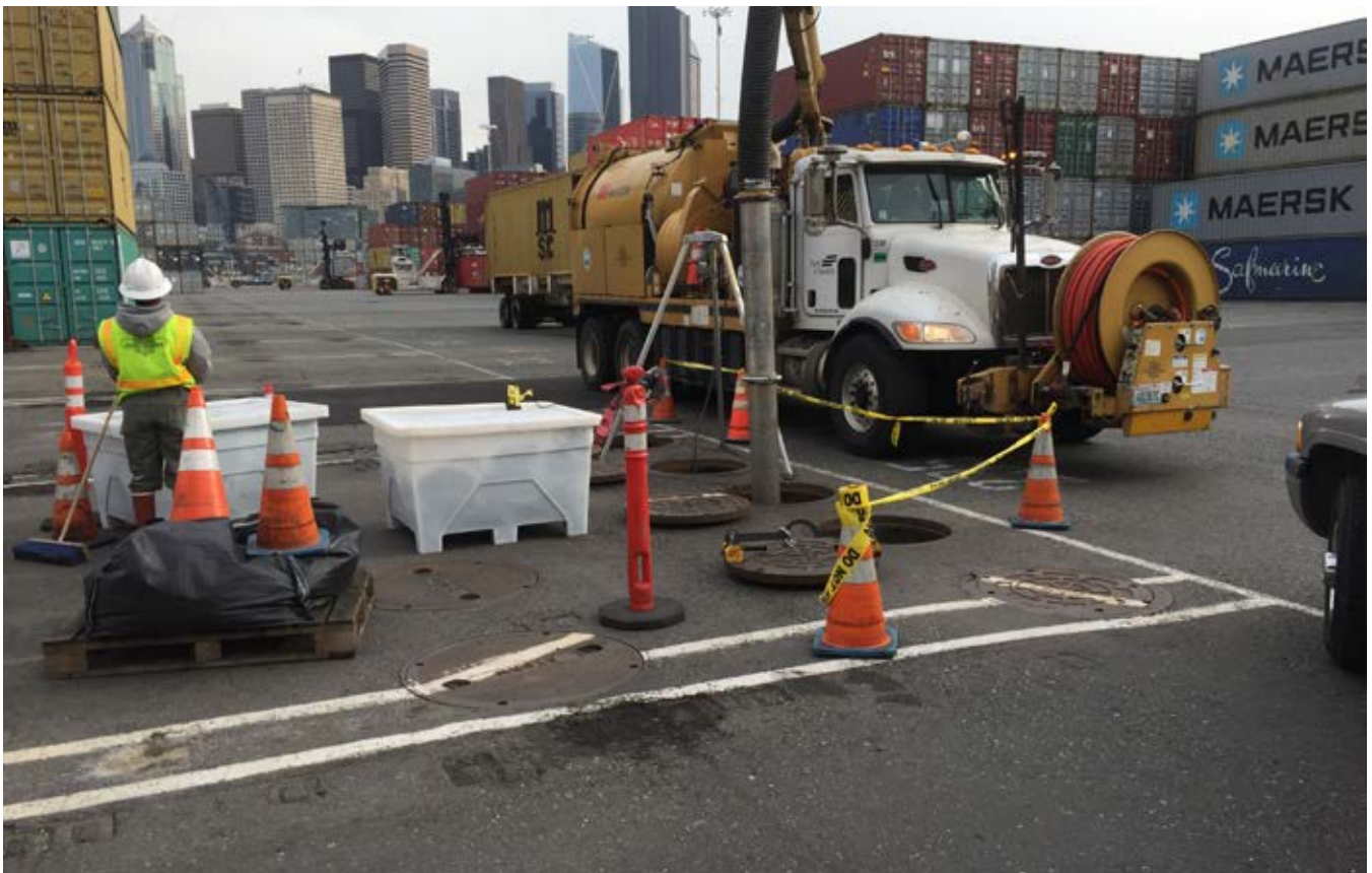
Replacing stormwater treatment media in vaults at Terminal 46
